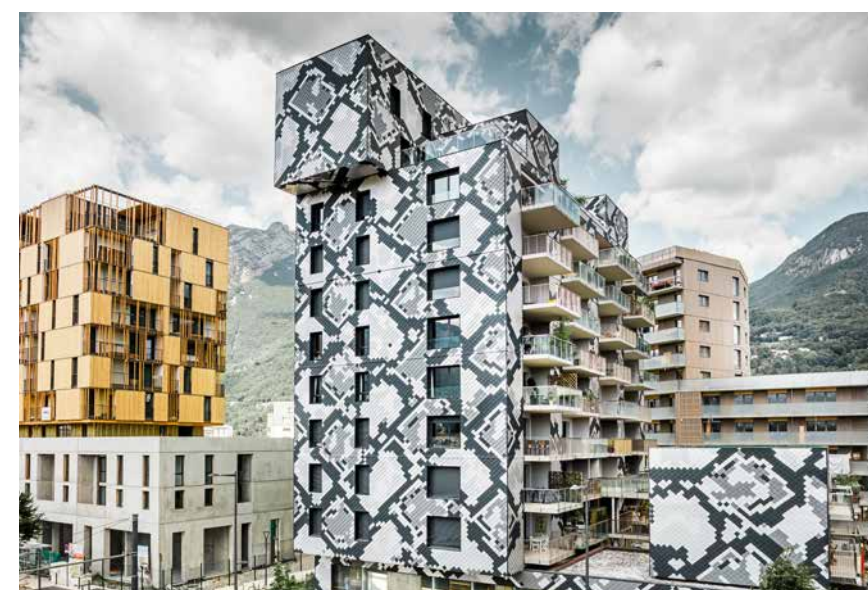
LE PYTHON GRENOBLE: RHOMBOID FAÇADE TILE 20 × 20 IN P.10 ANTHRACITE, P.10 LIGHT GREY, PLAIN ALUMINIUM AND METALLIC SILVER
