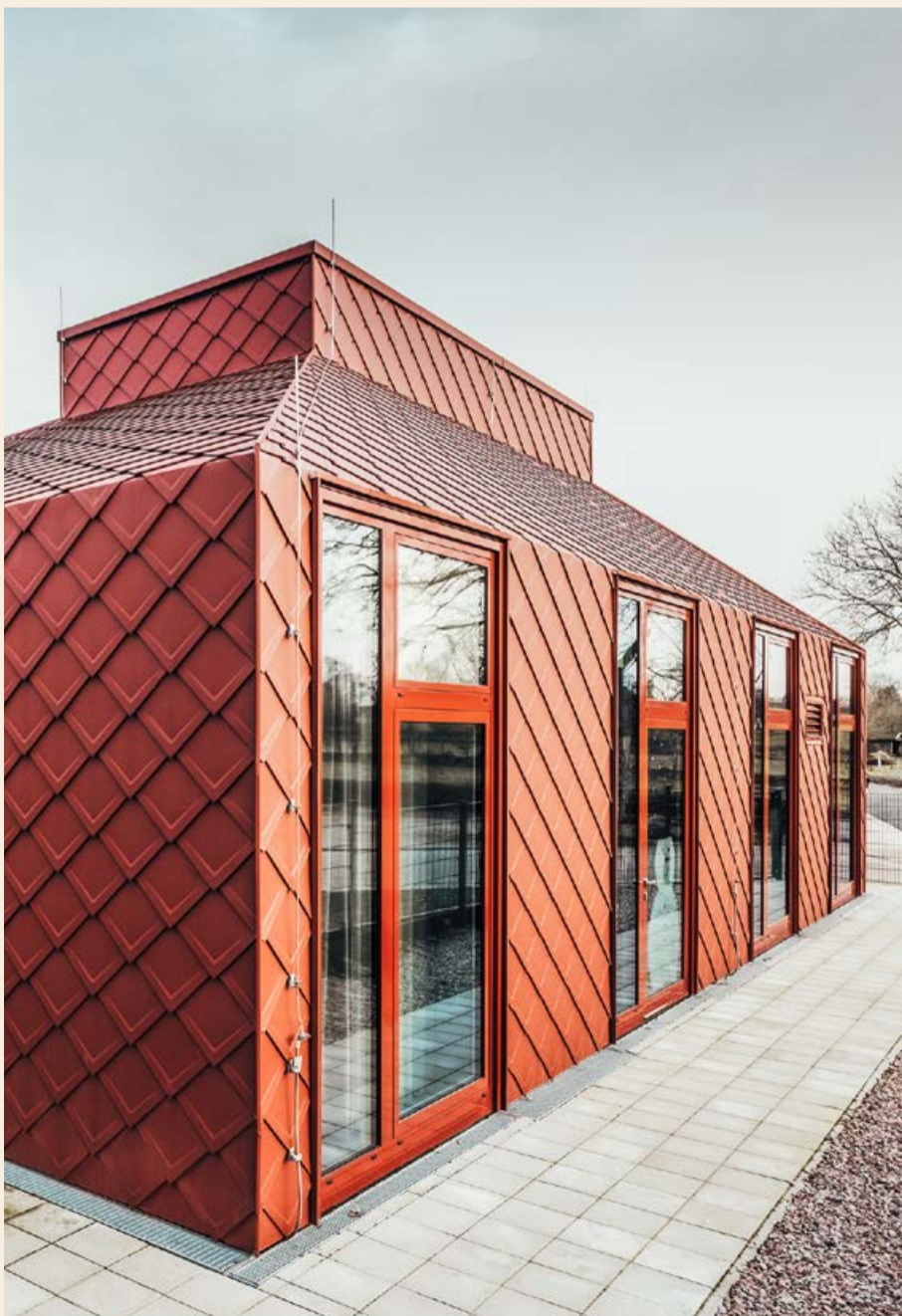
Object: day care centre, Hennstedt Product: rhomboid roof tile 44 × 44 Colour: P.10 oxide red ● Object-related individual solution Architecture: Jebens Schoof Architekten BDA, Heide
